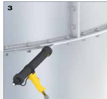
Seal the flanges on the outside.
