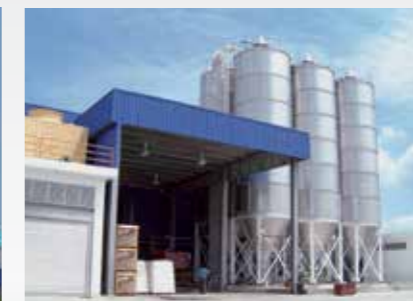
6 Stanriv® silos in Malaysia.
